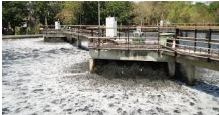
SLUDGE DIGESTION TANK
