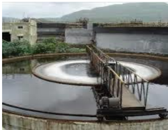
PRIMARY SEDIMENTATION TANK
